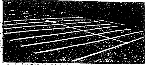
PVC ribs laid out and ready to assemble
