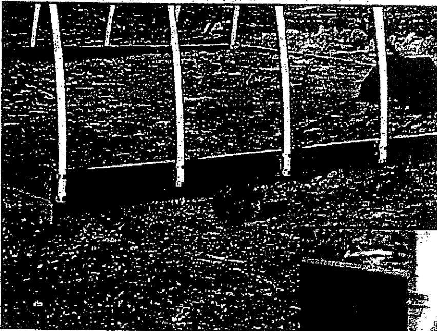
The PVC ribs are attached to the base boards
